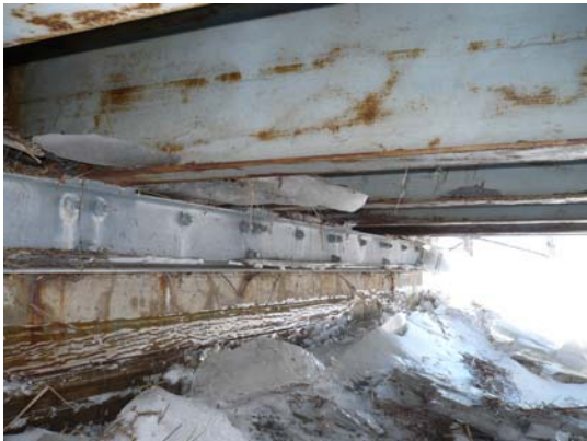
FIGURE 2: Channel added at beam ends for additional support.
