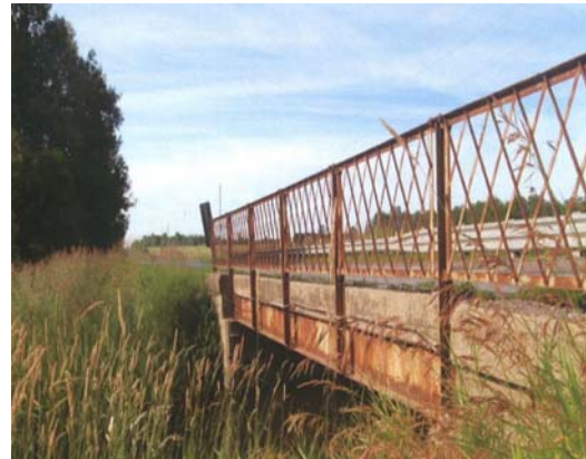
FIGURE 3: Inferior barrier wall.
