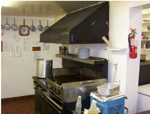
Before and After shots of commercial cooking operation – charred wood was found when old system was removed – new system (on the right) is in compliance with NFPA 96 – stainless steel hood, proper clearances from combustible surfaces, adequate exhaust and fire suppression system.
