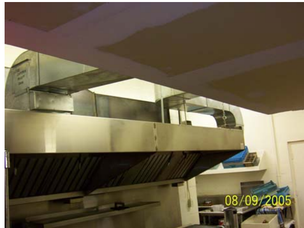
Before and After shots of commercial cooking operation – charred wood was found when old system was removed – new system (on the right) is in compliance with NFPA 96 – stainless steel hood, proper clearances from combustible surfaces, adequate exhaust and fire suppression system.
